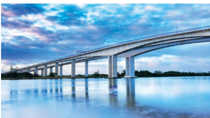
Monitor infrastructural deterioration in bridges
