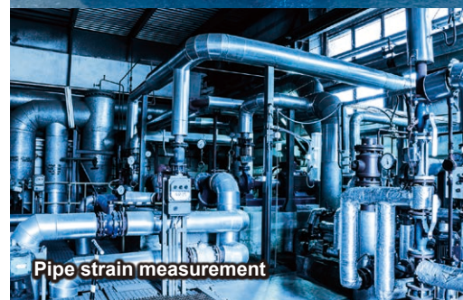
Brake and pipe strain measurement
